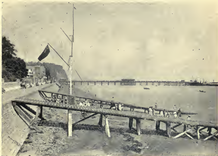
The Pier, Penarth.
